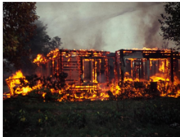
Former Church Office Removed in Practice Burn by SC Fire Dept.
